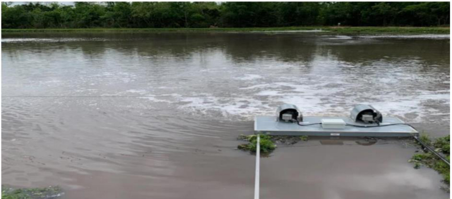
Installed 5 Stainless Steel Lagoon Masters and SewperRx Microbial Blend
